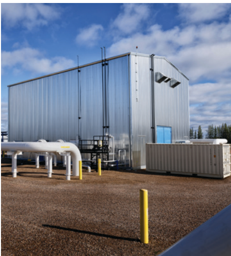
Example of a compressor station
